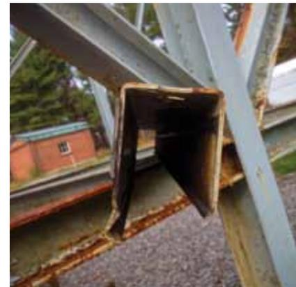
**ABOVE** They just wore out from use! One of the broken rails from the moveable roof protecting The Planetary Society All-Sky Optical SETI telescope in Harvard, Massachusetts. The worn-out rails were replaced and the roof is operating better than ever.
